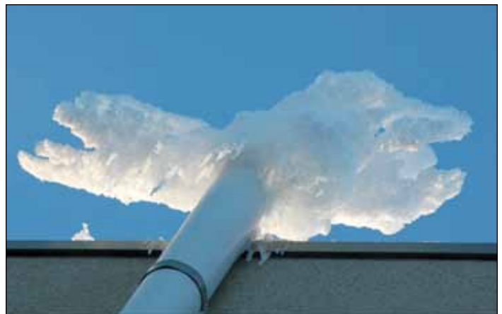
Figure 1 Frost covered radon vent in Winnipeg
