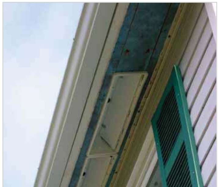
Figure 4 VSVs Installed. Blown closed. These first full-scale valved soffit vents are “working mockups” made from plastic window planters with light “corroplast” valves. They proved too noisy despite having soft rubber bumpers.
