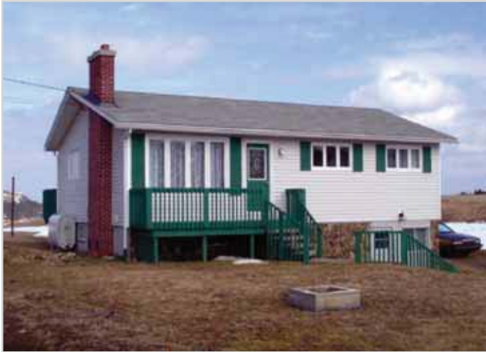
Figure 2 Pouch Cove House. Looking north at the front of house; chimney on east end. House plan is 26 x 36 ft. The roof sheathing is tongue-and-groove boarding, probably air-leaky especially where protruding over the gables.
