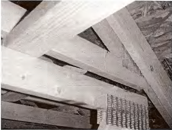
Figure 11: These piggyback trusses are not supported at the bearing point.
