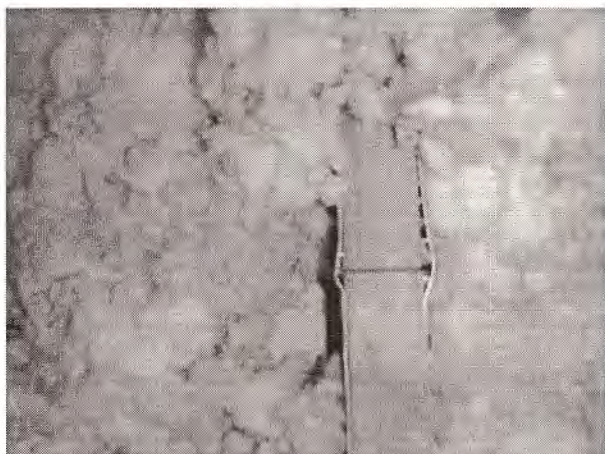
Figure 5: Compression buckling of connector plate on truss that was bent during installation (left).
