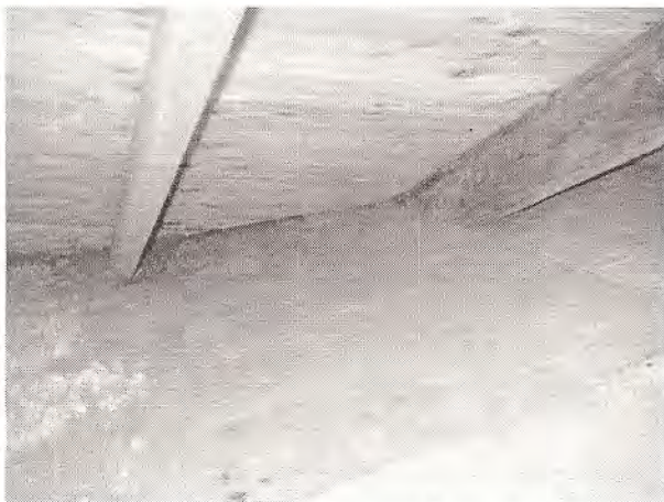
Figure 12: These rafters bear only on-roof sheathing in between trusses.
