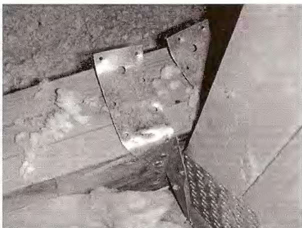
Figure 10: All nail holes should be filled in metal hanger brackets.
