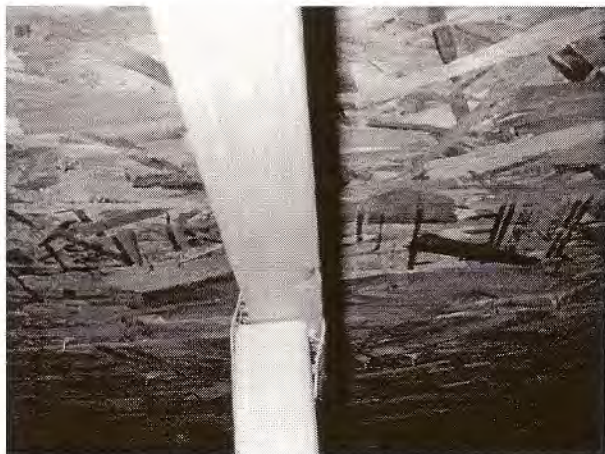
Figure 4: Metal connector plates loose strength even when pulled only part way out.
