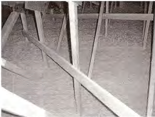
Figure 8: CLR is not effective when applied to trusses that do not have similar web patterns.
