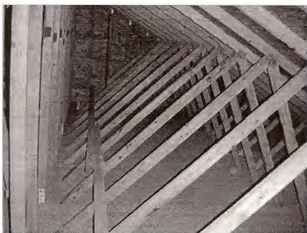
Figure 9: CLR should be roughly centered in span of web member.
