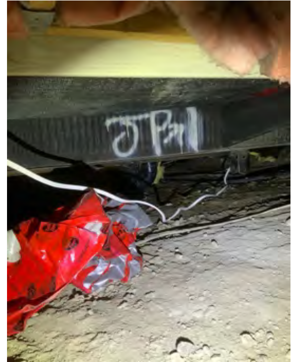
Wire should be secured to framing.
