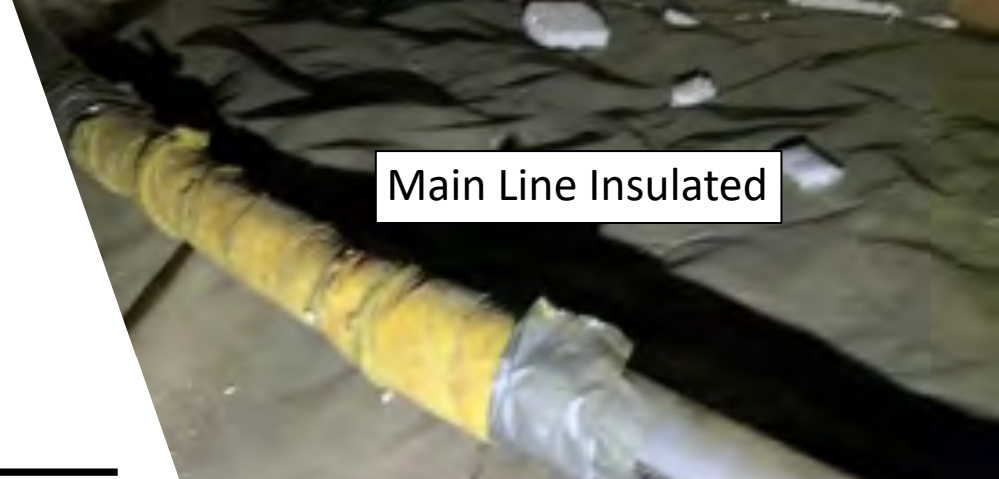
Main Line had heat tape Installed and connected
