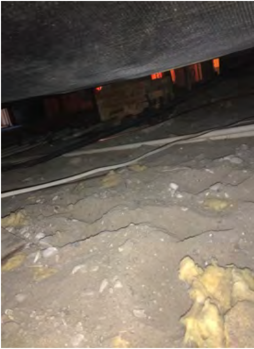
Wire should never touch the ground.
