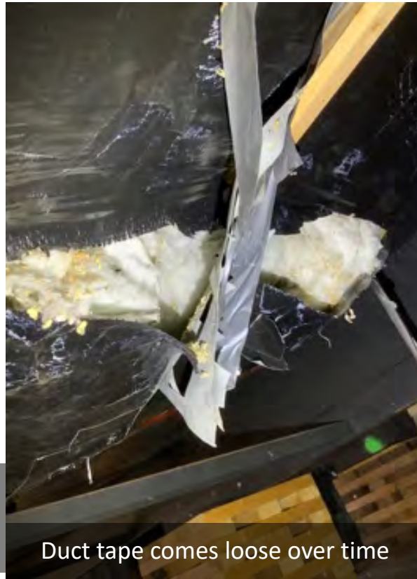
Tuck tape loses it's stick over time and rodents eat it
