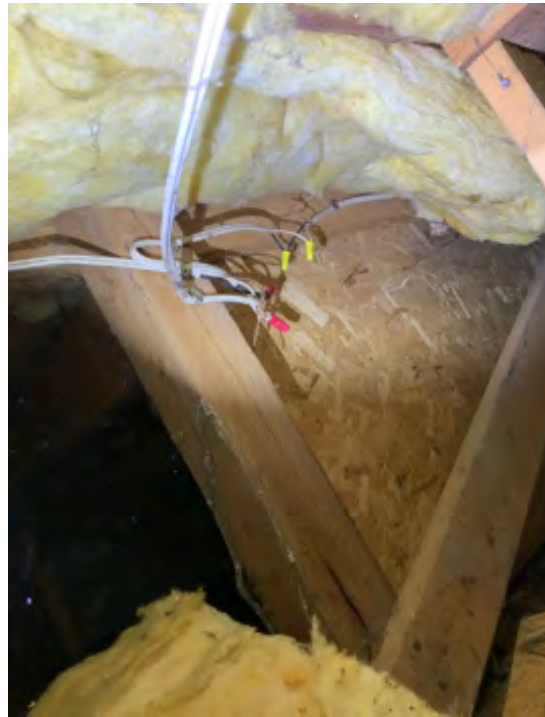
Open splice maybe a sign of DIY install.
